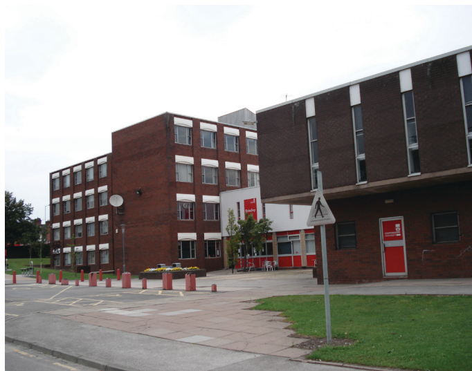
Brindley Building: Business School, Staffordshire University
